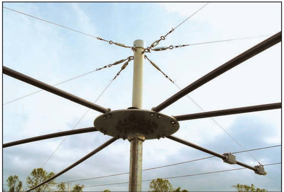
Figure 7—The guy wire center post, turnbuckles, and hub. Note the conduit boxes at the lower right. These serve as feed line junctions to the driven elements. The feed line and phasing line pass through the fiberglass support arm.
